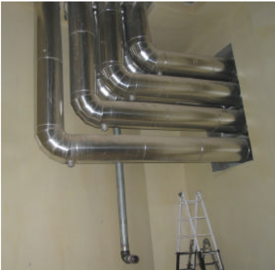
(b): The pipe fitted to the condensate cleaning port of Engine # 1 with a flow regulating valve
