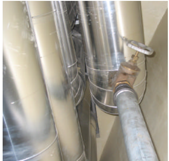
(b): The pipe fitted to the condensate cleaning port of Engine # 1 with a flow regulating valve
